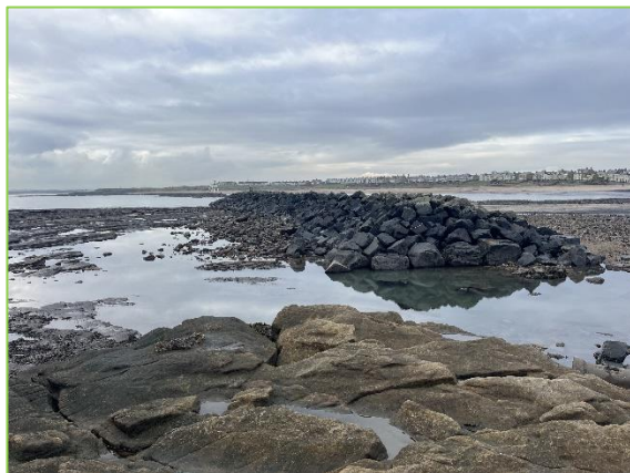
North breakwater in Newbiggin Bay in overall good condition (/3601C14)
