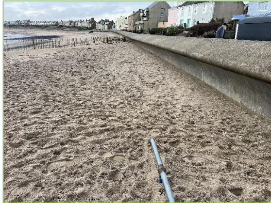
High Beach level to the north of the recurved wall partially submerging picket fencing (/3601C07)
