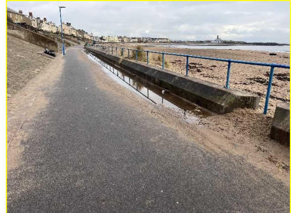
Block promenade drainage scuppers (/3601C08)
