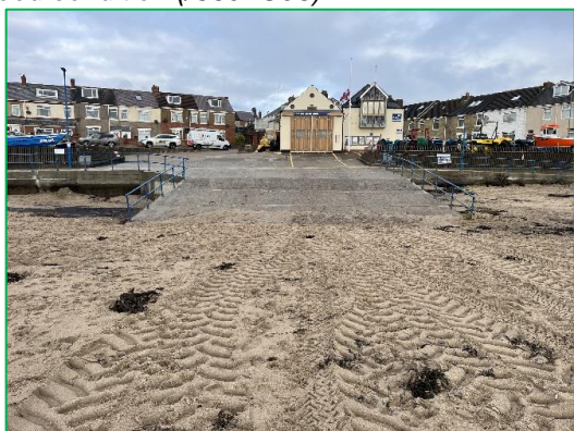
New concrete access ramp constructed 2022 (/3601C06)
