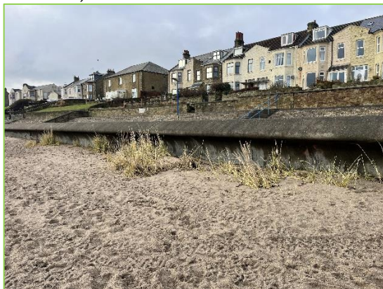
High Beach level to the south of the recurved wall, dune formation fronting the seawall (/3601C07)
