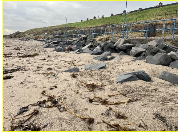
Some localised rock displacement but generally in good condition (/3601C08)
