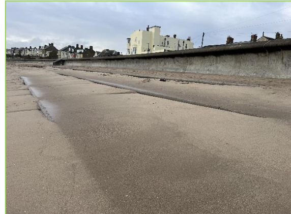
Lower beach levels in the centre of the bay exposing stepped apron (/3601C07)
