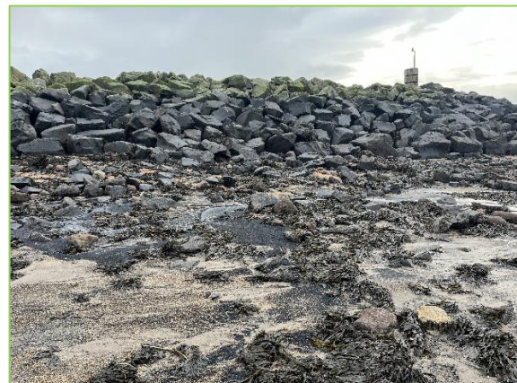
Smaller rocks displaced across the foreshore on both the seaward and landward aspect (/3601C14)
