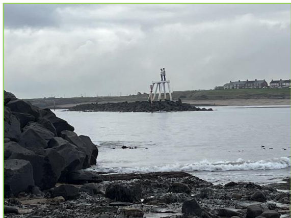
Detached breakwater in central Newbiggin Bay remains in good condition (/3601C16)
