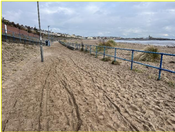
Large volumes of deposits on the promenade to the south of the bay likely due to the recent stormy weather (/3601C08)
