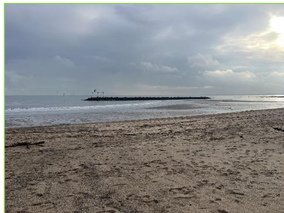
Salient/tombolo developed in lee side of the detached breakwater (/3601C16)
